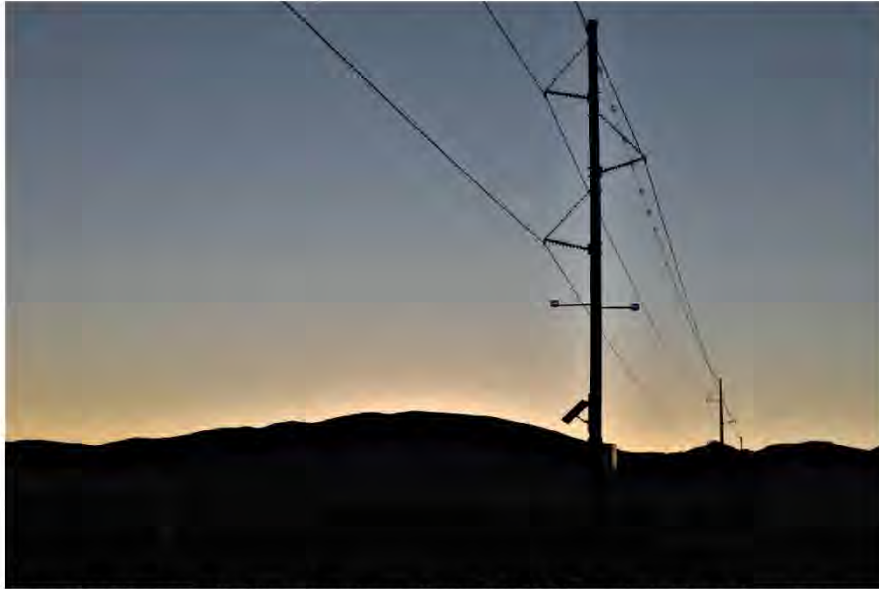
Figure 2. The Avian Collision Avoidance System (ACAS; purple lights on tower) uses ultraviolet (UV) light to illuminate power lines at night to reduce the risk of avian collisions. ACAS lights are faintly purple because they primarily produce UV light that is invisible to people.
